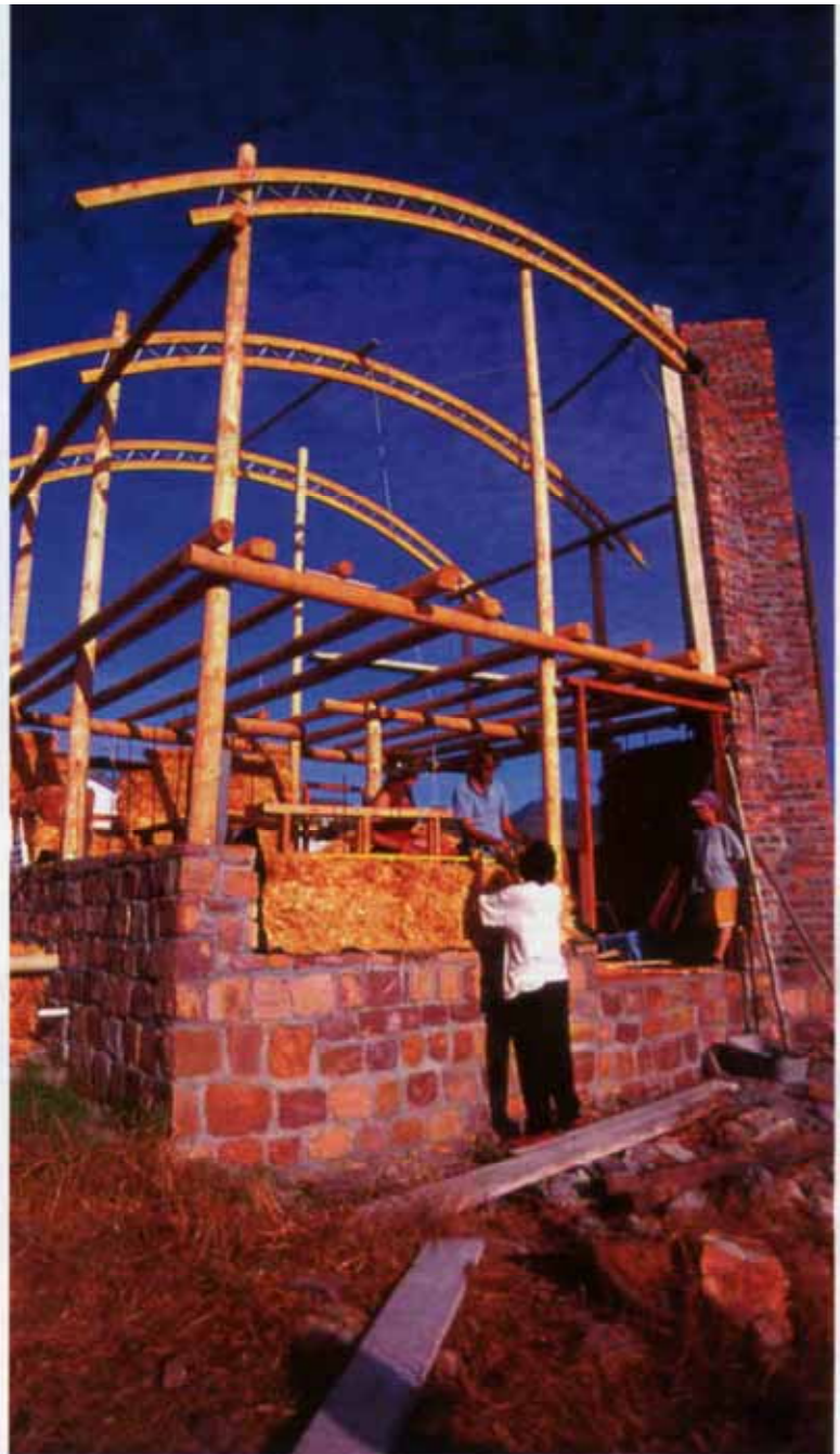
The photographs on this page show a holiday house in Scarborough which features a pole framework with stone walls and straw bale infill. Design: Eco Design Architects
