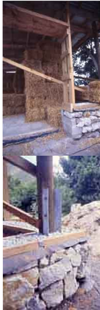
Pole brackets & garage door frame attachment
